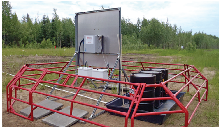
Solar Sipper installation with bovine protection
