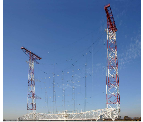
Short-wave curtain antenna station
