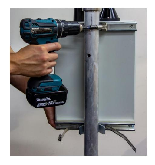
5. Adjust the position of the rails in relation to the mounting pole so that the pole is located at the center of both rails, using a spirit level to ensure the instrument is correctly leveled.
