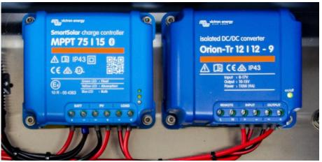
The solar regulator has been pre-configured to protect the battery from continuous discharging and charging cycling. Should the battery voltage drop to below 11.1V, the regulator will shut off supply to the DC/DC converter and subsequently to the load until the voltage recovers to above 13.1V.
