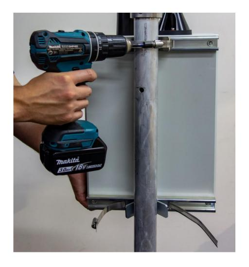
Adjust the position of the rails in relation to the mounting pole so that the pole is located at the center of both rails, using a spirit level to ensure the instrument is correctly leveled.
