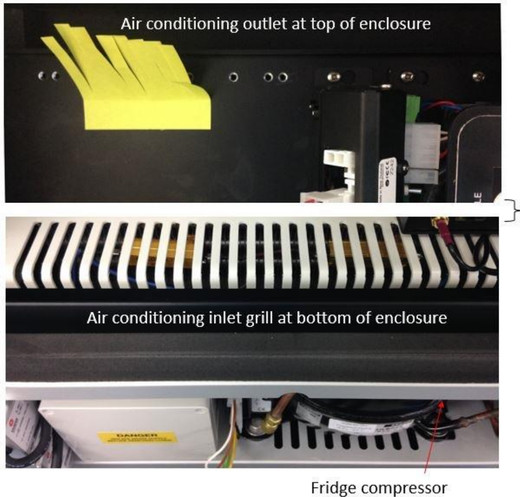
Figure 0-20 Air-conditioned air is constantly circulated in the AQM 65 enclosure. Air comes in to the enclosure at the top and exits through vents at the bottom
