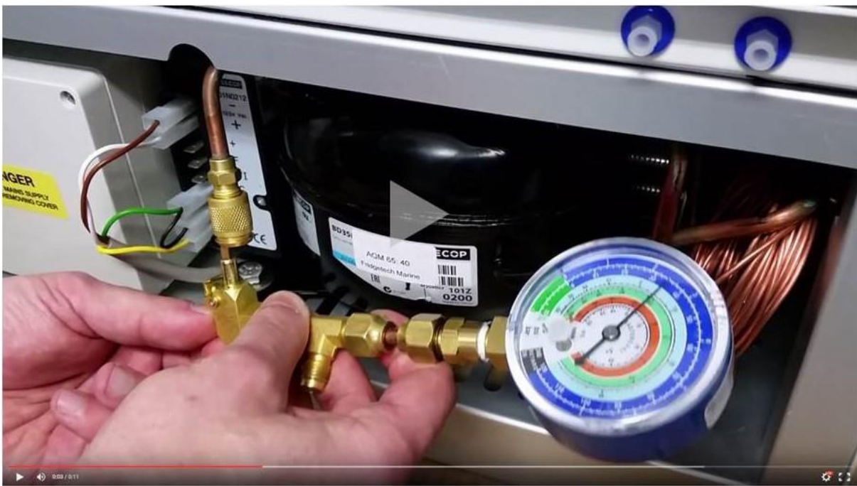
Figure 0-38 The pressure gauge pushes in to the fitting on the compressor inlet
